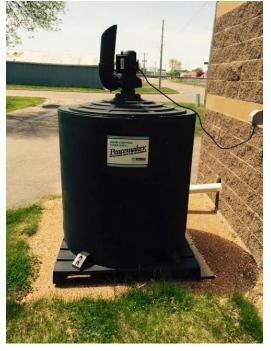
PEACEMAKER® Dry Air Scrubbers provide two stage chemistry for the control of odors from hydrogen sulfide (H<sub>2</sub>S), mercaptans, ammonia, amines and other odors generated in wastewater collection and treatment systems. They are easy to use, effective and economic and have no maintenance.
