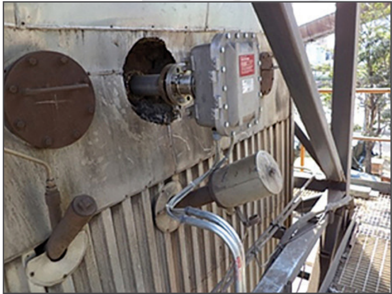
Flue gas monitoring at a cement plant
